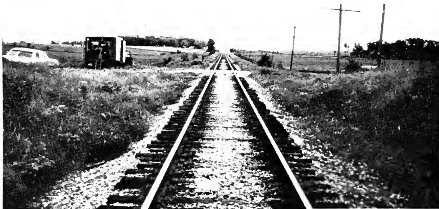
Fig. 1—Test location for study of rail anchorage forces on continuous welded rail.
